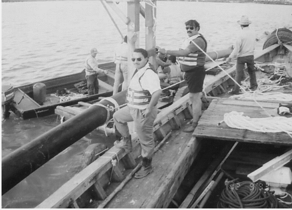
Pulau Besar (Melaka) submarine pipe sinking process guided by Virum from Finland. This is on our usual tug boat used to launch the pipe into sea.
